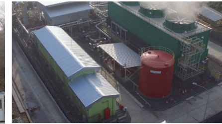
B Dieng Small Scale Geothermal Power Plant, 12.6 MW Wonosobo, Indonesia
